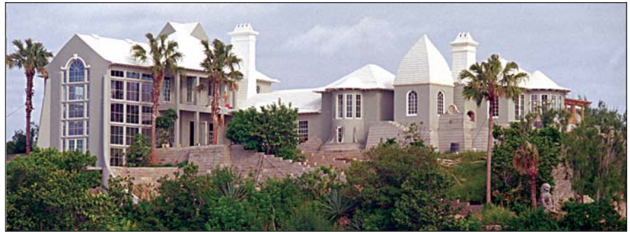
This sprawling 11,000 sq. ft. mansion, on nearby Agar's Island, features 170 Atlantic fixed and casement windows with Super Spacer. To view additional Atlantic Window projects, visit www.atlanticwindows.com .
