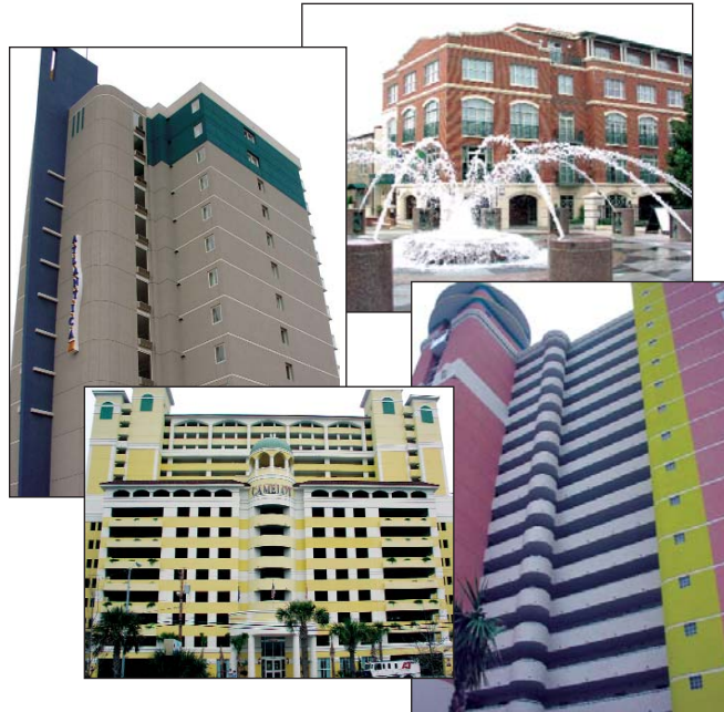
Coastal Glass installations at Carolina resort hotels: (clockwise from top) Vendue Range, Baywatch, Camelot and Atlantica.
